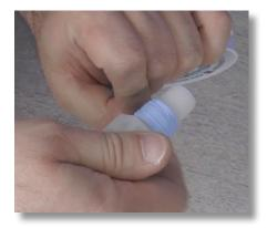
**Step 31:** Take the thread seal tape and wrap it around the threads of the Injection Valve for the necessary size -3/8" or  $\frac{1}{2}$ ".
