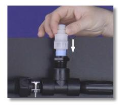
**Step 9:** Reinstall the Injection Valve into the installation saddle, hand-tight.
