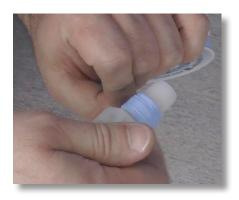
**Step 31:** Take the thread seal tape and wrap it around the threads of the Injection Valve for the necessary size -3/8" or  $\frac{1}{2}$ ".
