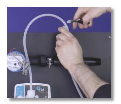
**Step 42:** Grab the rigid polyethylene discharge tube connected to the discharge valve. Using diagonal pliers, cut the tube so that it runs comfortably from the discharge valve to the injection valve.
