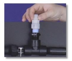
**Step 41:** Install and hand tighten the Injection Valve into the installation saddle or tee in the supply line. Do not overtighten.
