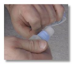
**Step 40:** Take the thread seal tape and wrap it around the threads of the injection valve for the necessary size; either 3/8 or 1/2 inch.
