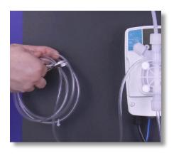
**Step 67:** Using the diagonal pliers, cut the tube so that it is long enough for the chemical bleed off to go into the bucket or stock tank.
