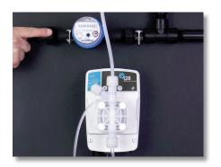
**Step 9:** If the **e128** works individually, it is time to test the water meter.
