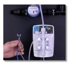
**Step 4:** If the issue continues, inspect the connection to the water meter to see if it is loose or disconnected.
