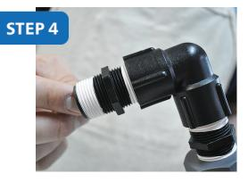
Attach the other **2**" **nipple** to the other side of the **elbow**.
