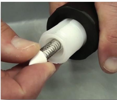
**Step 9:** Then carefully pry the check valve assembly (Part #: MPDI122) down and out of the stem. Discard the old check valve seal and assembly.
