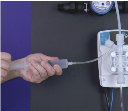
**Step 58:** Using the syringe kit, slide the syringe onto the air bleed barb and draw the plunger back. Chemistry should enter the syringe. Eject the chemistry from the syringe into the chemical bucket.
