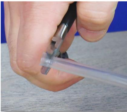
**Step 20:** Look at the end of the tube. If the tube's end is flared, use the diagonal pliers or cutters to cut the flared portion off.
