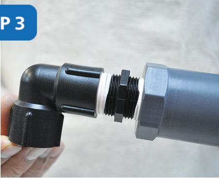
Thread the **3/4" female to female elbow** to the **nipple** and hand tighten.
