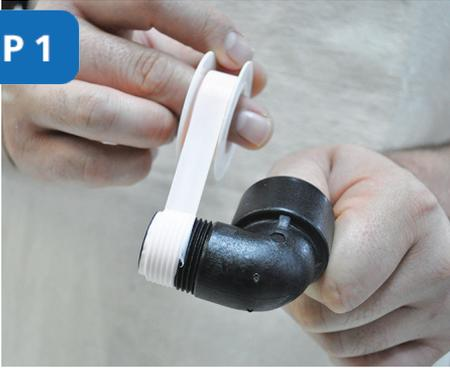
To begin, be sure to wrap all pieces with the **thread seal tape**, in a clockwise rotation, around the pipe threads. This will prevent the tape from coming off during assembly.
