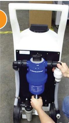
Attach the Dosatron unit and Quick Hook-Up Kit assembly onto the unit bracket.
